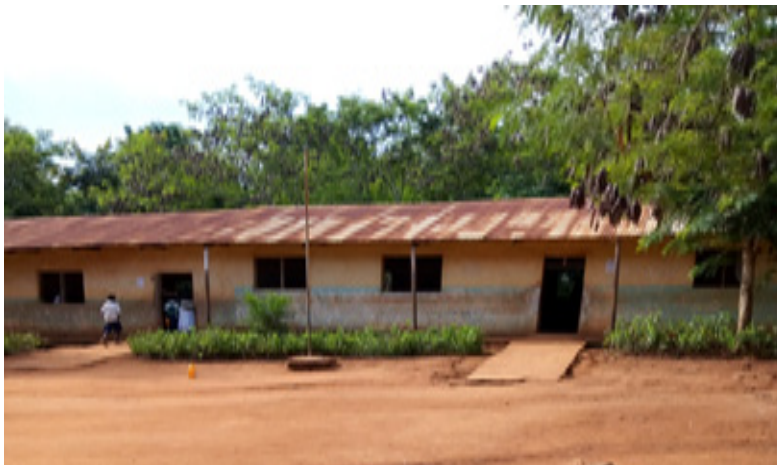
Field Photo showing Ramps in classroom entrance at school ‘Y’.
